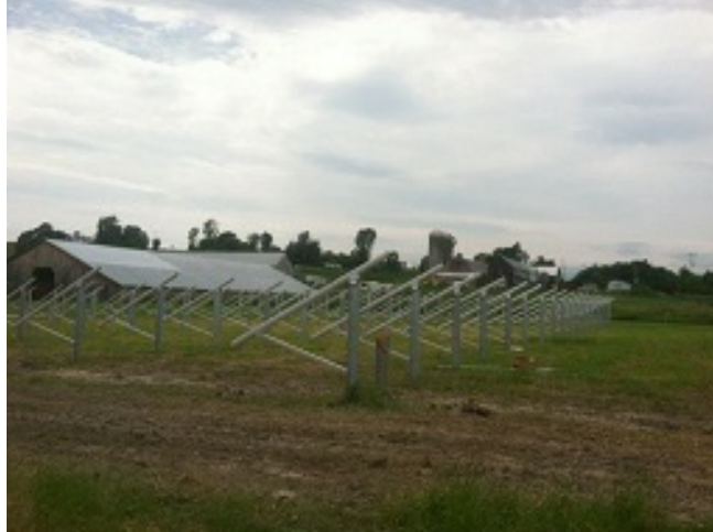
Installation underway at Misty Knoll Farm.
